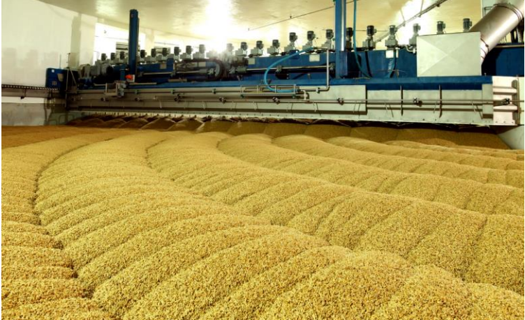
Image 1 + 2: Fans and motors are vital within Munton’s large-scale production process, by using Mitsubishi Electric’s Smart Condition Monitoring (SCM) system these are protected against unscheduled downtime.
